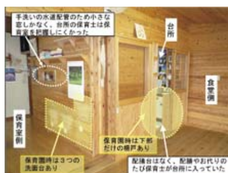
改善前 Before Improvement
